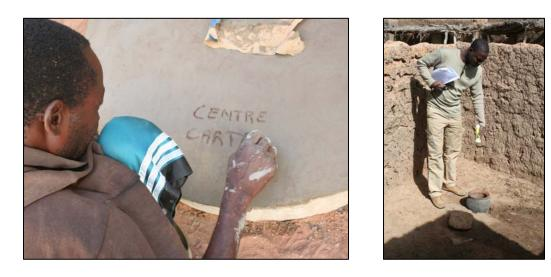
A mason (*at left*) finishes a latrine slab. At right, a traditional latrine is inspected during a latrine evaluation.
